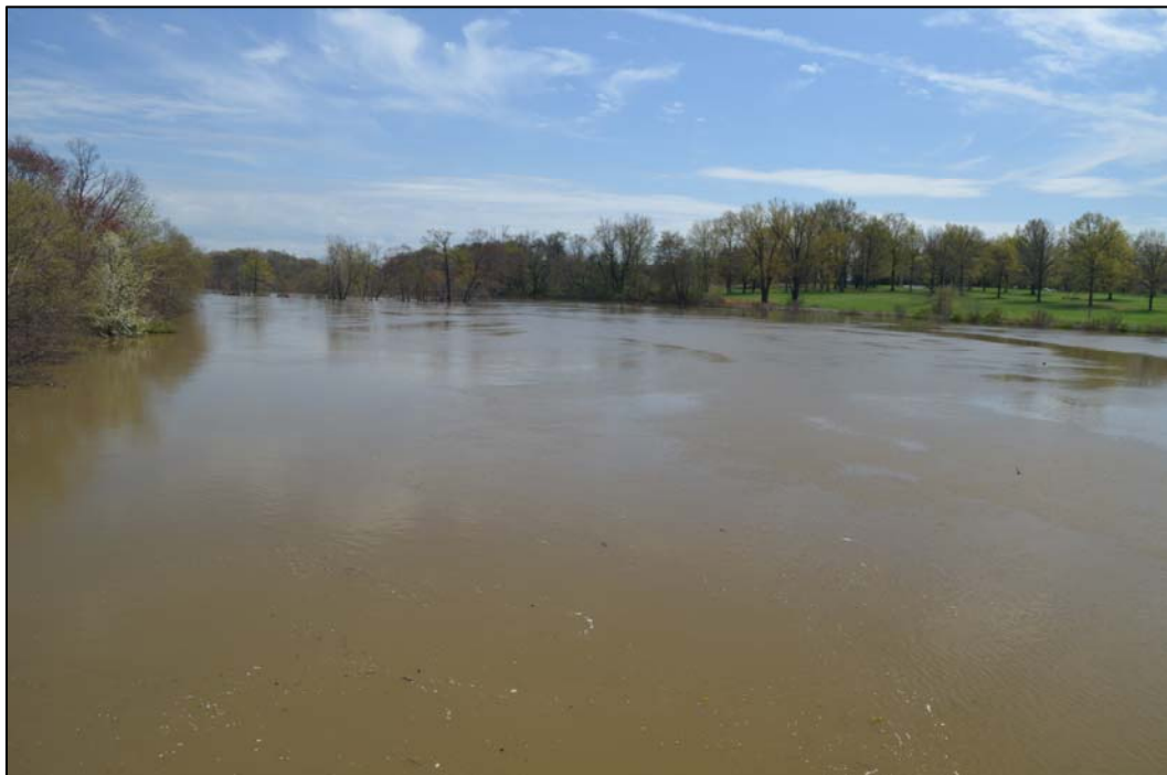
Photograph 4 – Upstream of U.S. Route 1 Bridge
