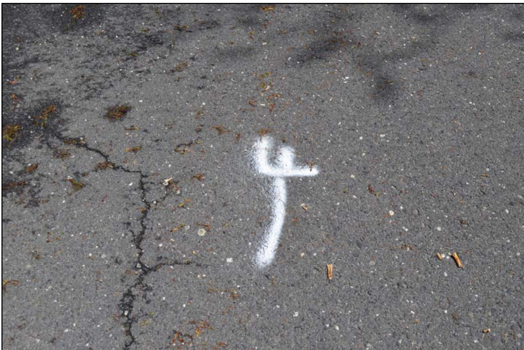
Photograph 14 – High Water Mark at Fieldston Road
