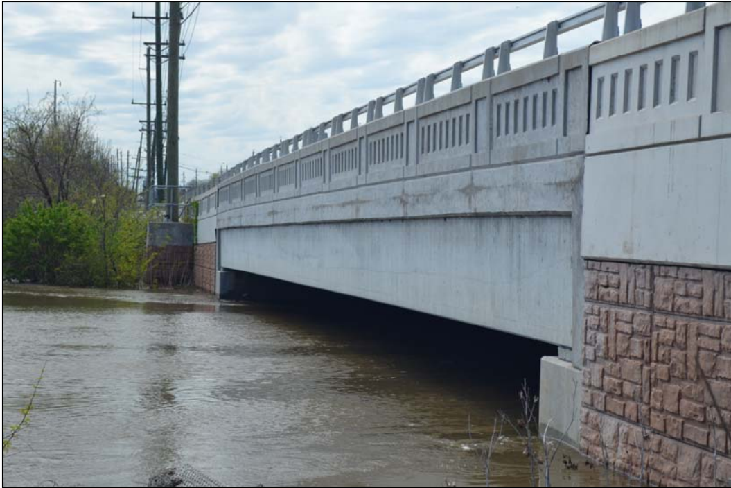
Photograph 5 – Upstream Face of U.S. Route 1 Bridge
