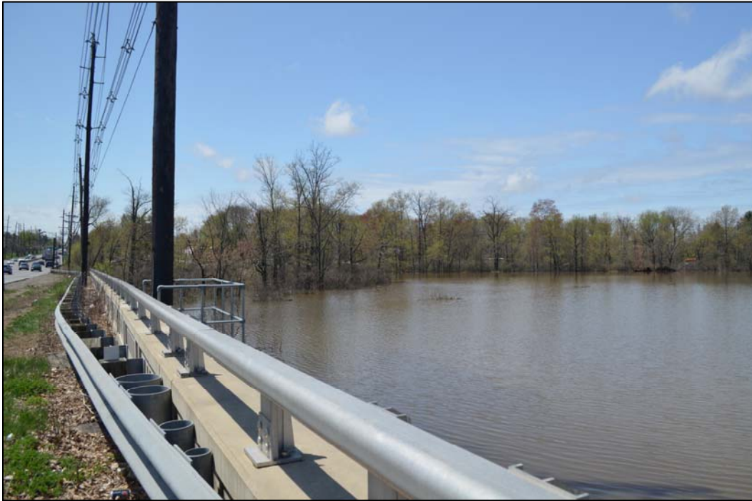
Photograph 3 – Downstream of U.S. Route 1 Bridge
