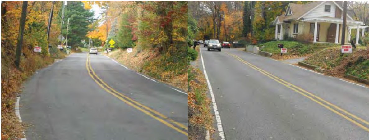
Figure 2 – Examples of Common Roadside Constraints on Cranbury Road
